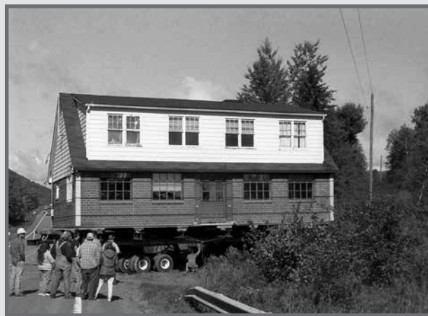
The Cole residence being moved in September 1991. DCEC.
