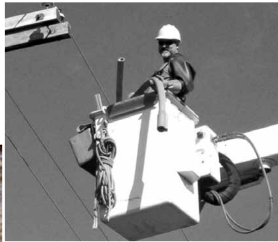
Left: Lineman Kim Armstrong in action.
