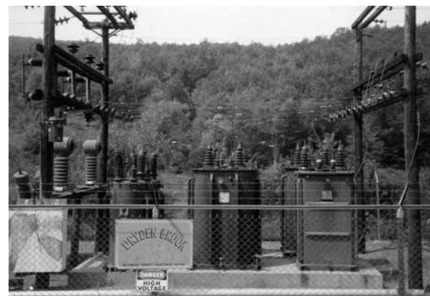
Dryden substation in 1978. DCEC.
