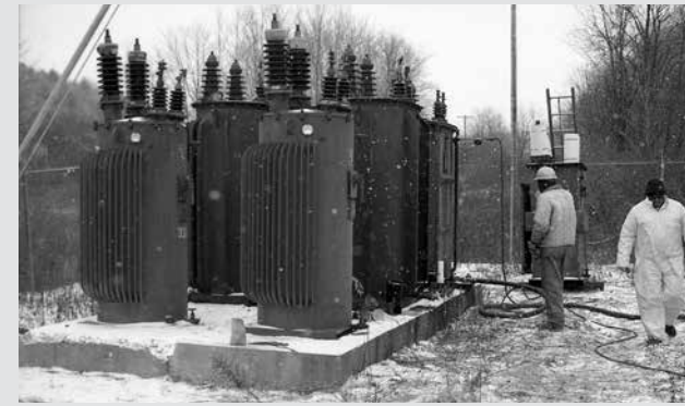
Transformers are removed, drained, and loaded for the start of their journey to El Salvador. DCEC.
