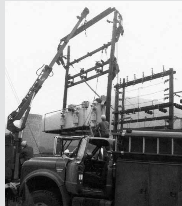
This pole became top heavy and broke, requiring a major repair to make it stable again. DCEC.
