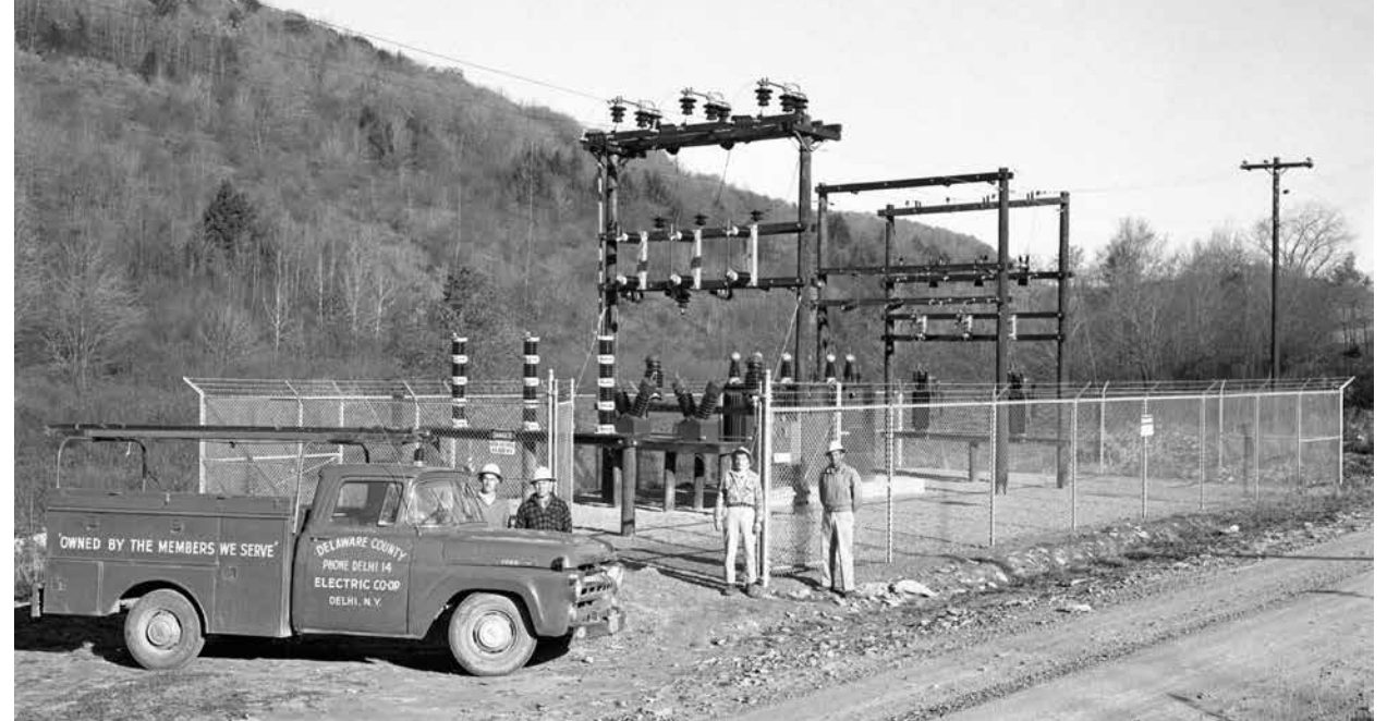
Walton substation, photographed in October 1958 by Bob Wyer. DCHA.
