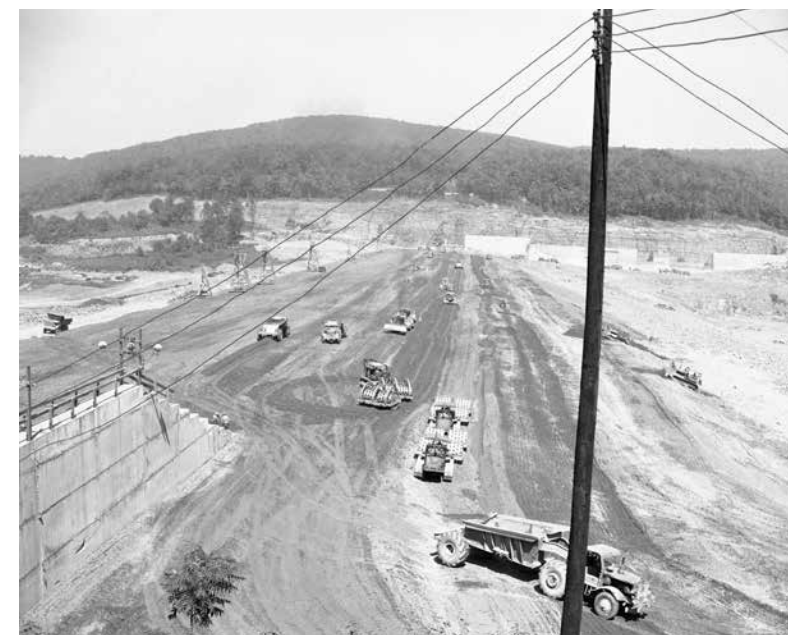
Top: Aerial view of the construction of the Downsville Dam, September 1949. PHOTOGRAPH BY BOB WYER, DCHA.
