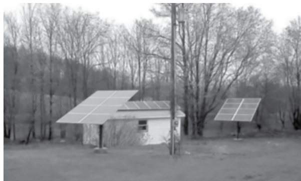
Solar panels, 2011. DCEC.
