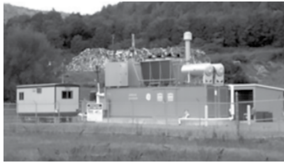
Delaware County Waste-to-Energy Project, 2012. DCEC.
