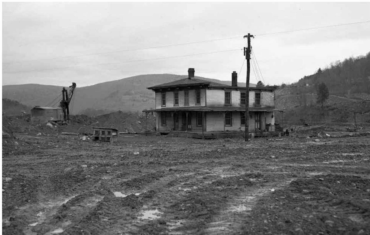
East Branch lines during the construction of the Pepacton Reservoir. DCEC provided temporary service during the construction for several businesses and for the engineering office. The buildings were ultimately demolished, and the lines relocated, when the reservoir was completed. These photographs were taken in May 1948. PHOTOGRAPHS BY BOB WYER, DCHA.
